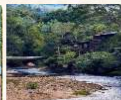
Kallar River & Hanging Bridge
